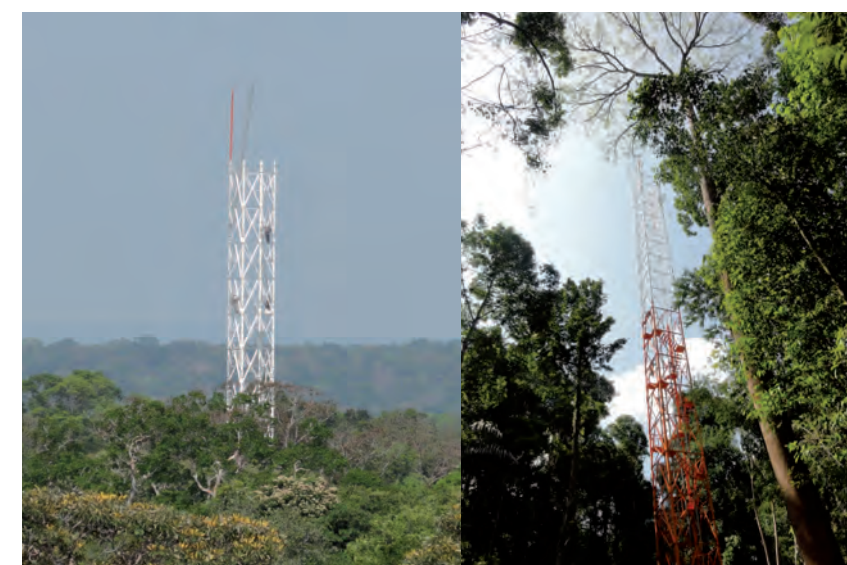
Figure 2: ATTO is steadily growing – here it reached about 100 meters.
