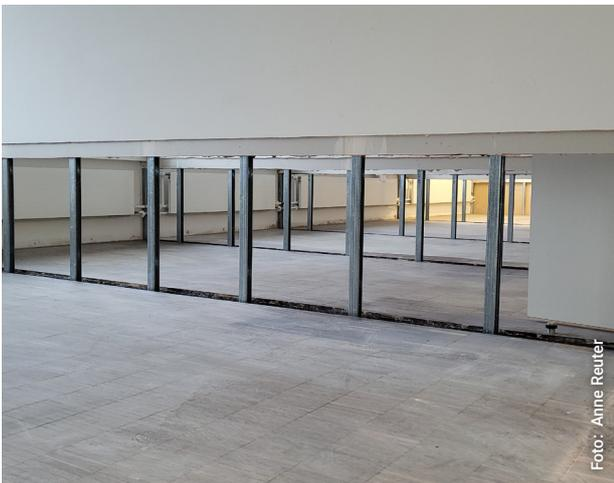
Freier Durchblick in die Nachbarbüros: Die feuchten Wände mussten 50 cm hoch abgebaut werden. | Unobstructed view into the neighboring offices: The damp walls had to be dismantled up to a height of 50 centimeters.
